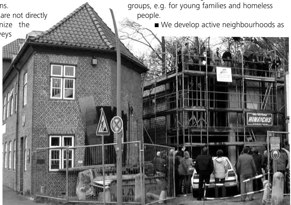
New building of the Lawaetz Foundation
