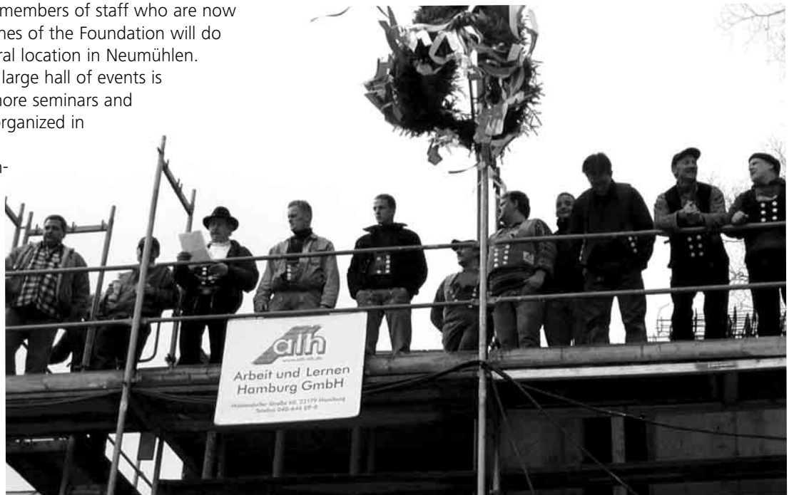
The topping out of the extension to the Lawaetz Foundation's
